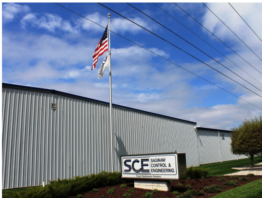
Saginaw Control and Engineering is located at 95 Midland Rd. in Saginaw Charter Township.
