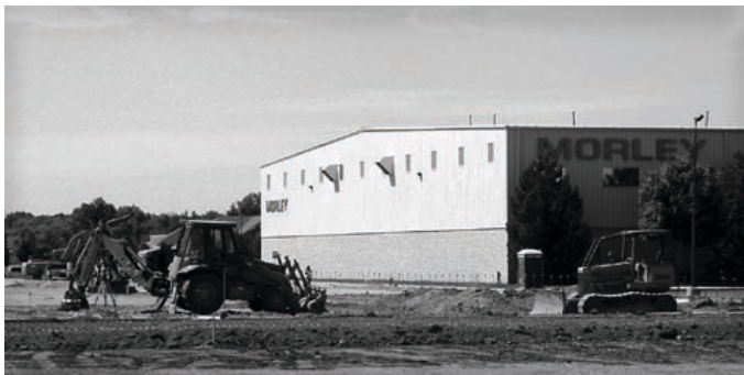
Construction at Morley Companies has already started.
