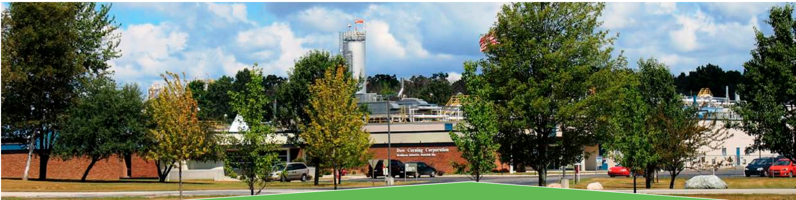
Above - Dow Corning Corporation Healthcare Industries Materials Site, a manufacturer of silicon-based materials for the health care industry, invested more than $2.5 million.
