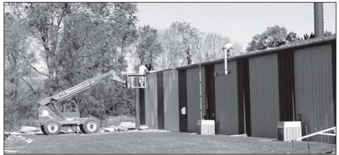
Allied Tool & Machine Co.'s expansion project included adding more manufacturing space.
