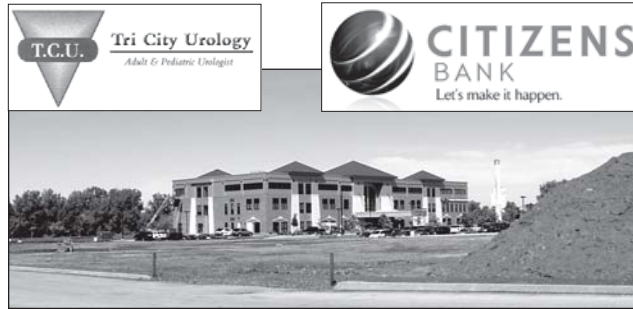
The Riverfront Medical Arts Condominiums will be located on S. Washington Ave. adjacent to MCVI.
